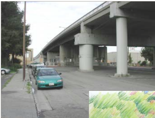
View of Transit Plaza and Rail Stop - before ...
